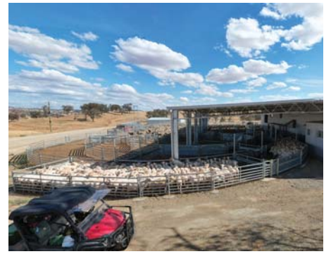
The new ProWay-designed shed and yards.
