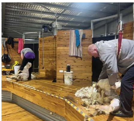
The new shed at Barrama that is based on the AWI Shearing Shed Design.
